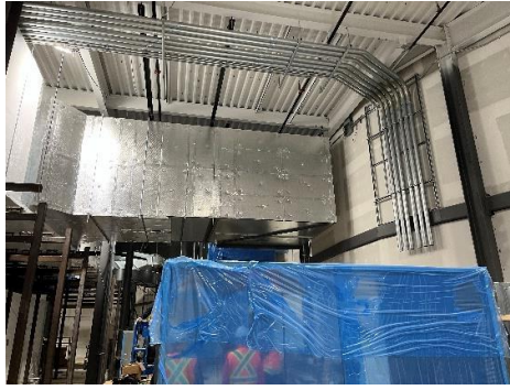
Smooth transitions, completed vapor retarder
