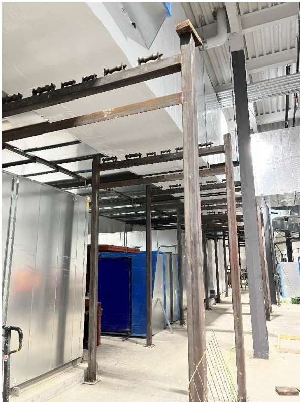
Flexible laminated pressure sensitive field-applied vapor barrier applied over board insulation
